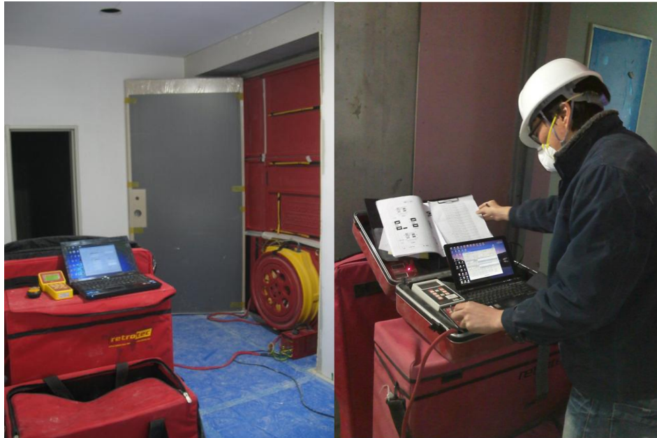
Fig. 1 Supporting photos of the air leakage test
