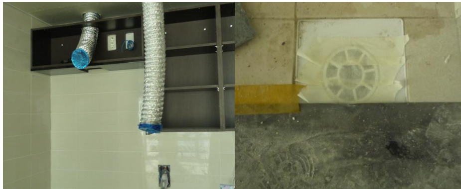
Fig. 2 Supporting photos of the temporary sealing
