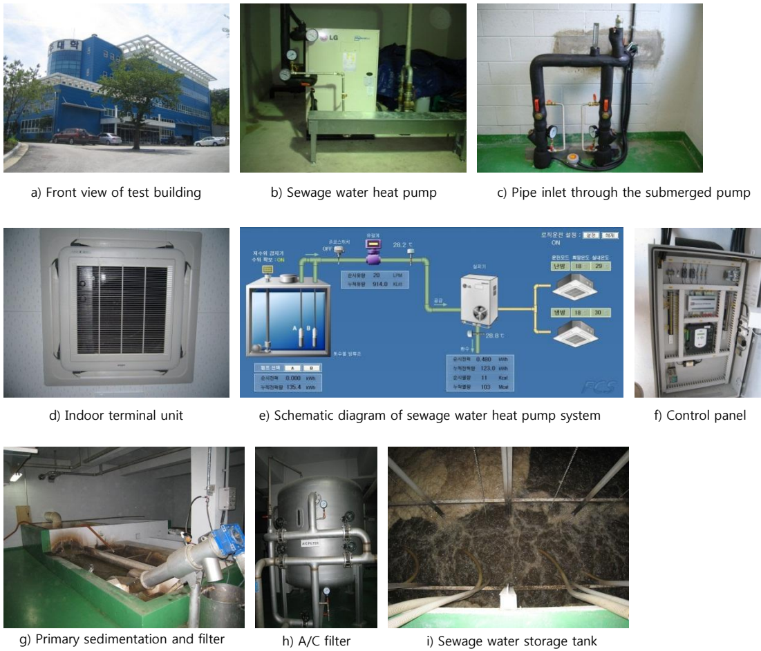
Fig. 1 Photos of pilot project system in test building
