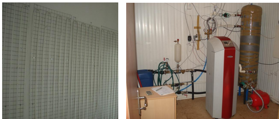
Fig.1 : (a) Wall heating serpentine (b) The investigated heat pump system
