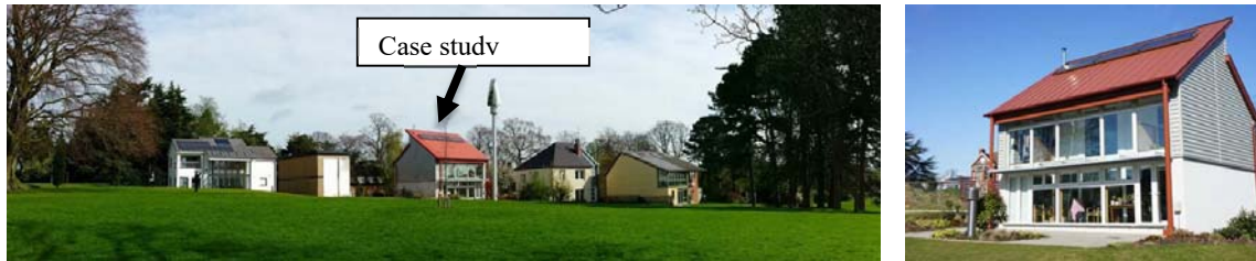
Figure 1: Location of the case study house and perspective view of its South and East facades
