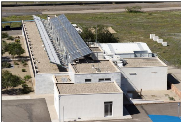
(c) Office building. View of the exterior
