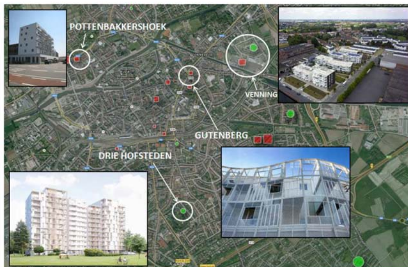
Figure 1: Overview of the demonstration sites in Kortrijk
