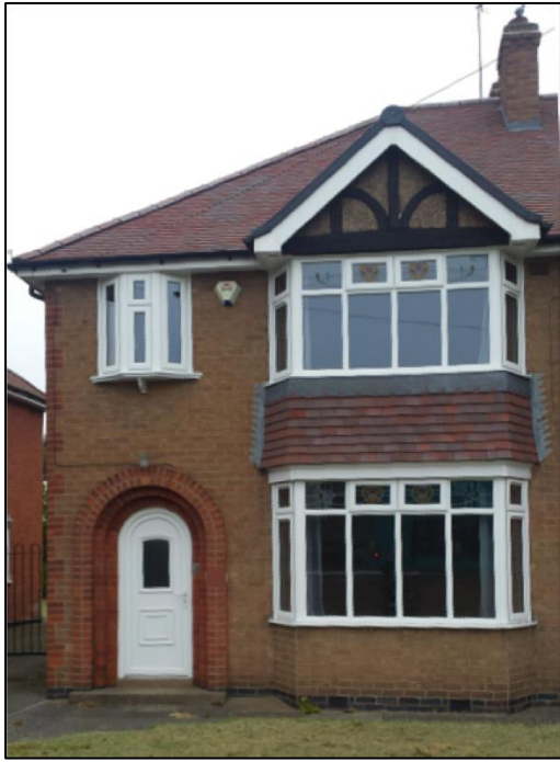
Figure 1. Photograph of the test dwelling.
