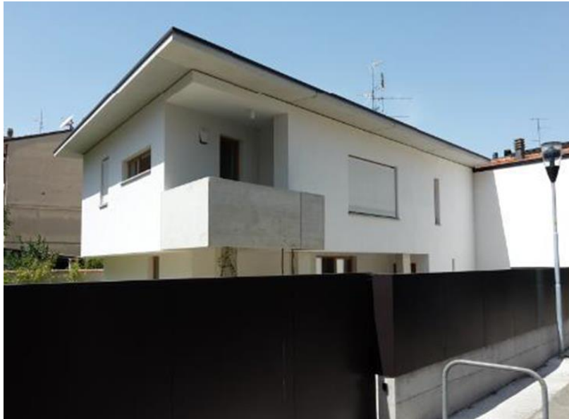
Figure 1: Nearly zero energy house in Modena, Italy
