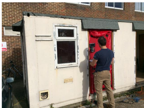
Figure 10 Setup of blower door (SW test)
