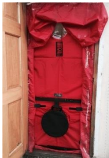
Figure 7 Setup of blower door
