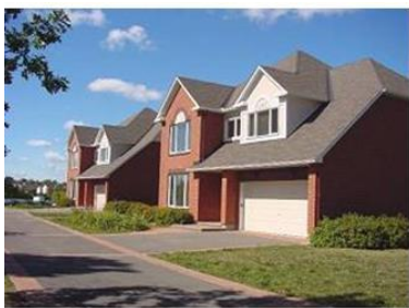
Figure 2. CCHT twin houses (left) and their characteristics (right)
