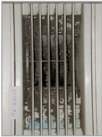
Figure 22: Hygroscopic bathroom exhaust unit, with protection grid
