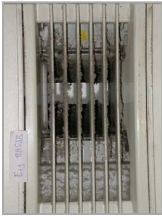
Figure 16: Bathroom humidity-controlled exhaust unit, with protection grid
