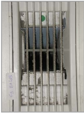
Figure 10: Bathroom humidity-controlled exhaust unit, with protection grid
