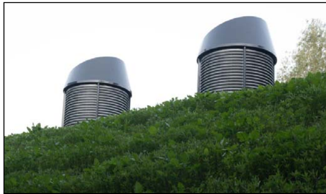
Figure 2: Prefabricated ventilators which utilize the Venturi effect. 4
