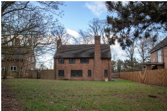
Figure 6: Back view of test building
