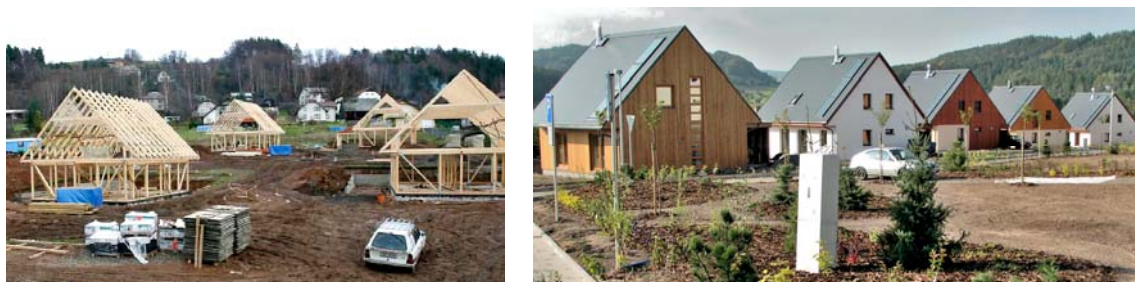
Figure 1 The studied buildings. Left – construction process. Right – completed buildings in 2007
