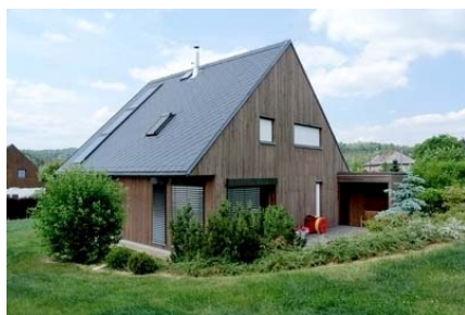
Figure 5 The building B in 2018
