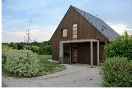
Figure 9 The building D in 2018
