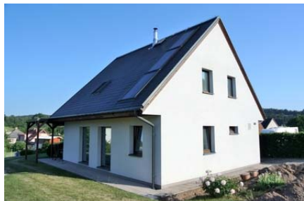
Figure 3 The building A in 2018
