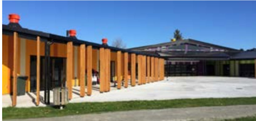
Roof mounted wind catchers
