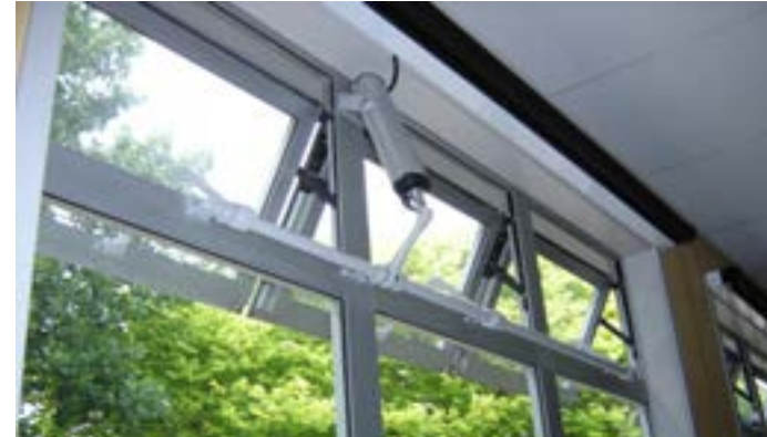
Opening high level windows
