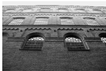
Figure 11 North elevation of the old factory
