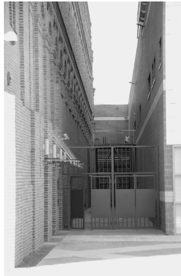
Figure 10 Passage between buildings
