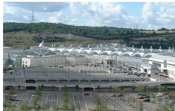
Figure 14 Bluewater with large naturally ventilated car parks and iconic ventilation turrets
