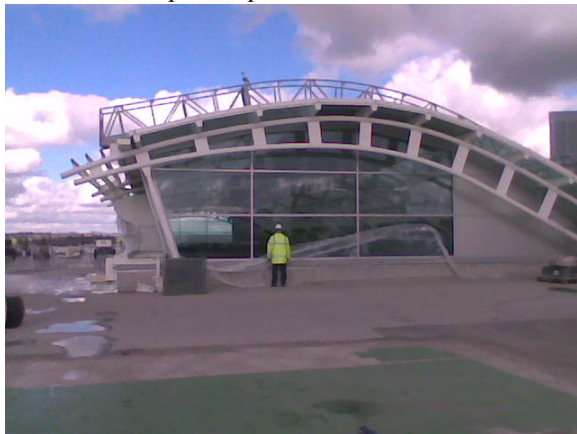
Figure 6 Roof turret in relation to Gull-wing roof
