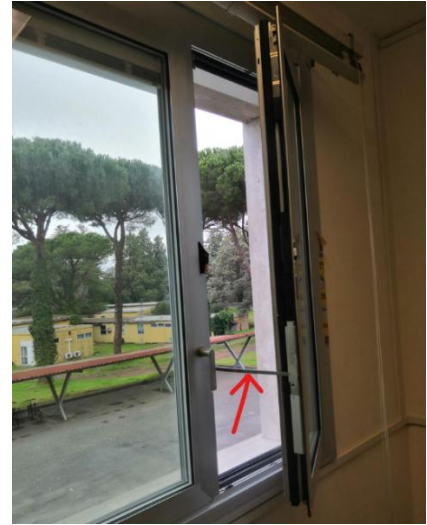
Figure 53: Front view of the new window, left, with the push-button indicated on the right sash; detail of the motorized chain to open/close the sash on the right. (Zinzi, Botticelli, Romano, & Agnoli, 2024)
