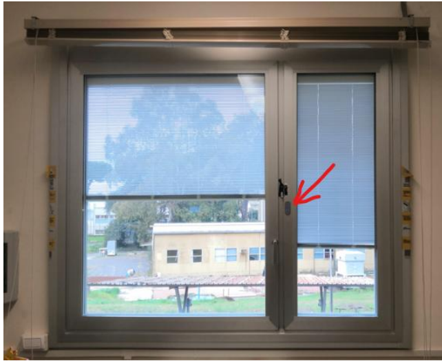
Figure 53: Front view of the new window, left, with the push-button indicated on the right sash; detail of the motorized chain to open/close the sash on the right. (Zinzi, Botticelli, Romano, & Agnoli, 2024)
