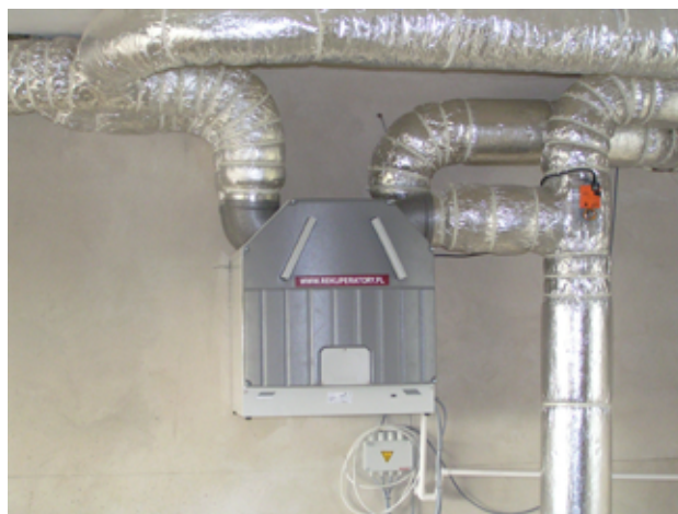
A ventilation heat exchanger. Source: Rekuperatory.pl, Poland
