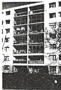
Fig.1. Test building with sunspaces
