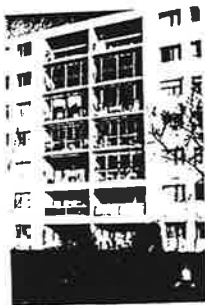
Fig.1. Test building with sunspaces
