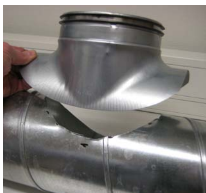
Figure 22 Collar saddle for in-situ tees [source: L.A.Matsson]
