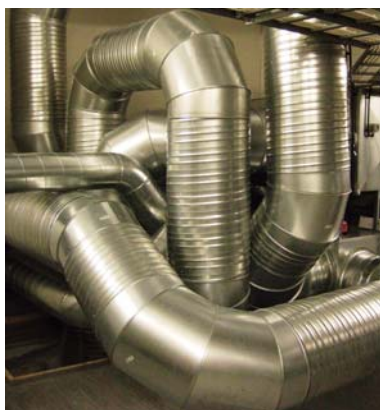
Figure 17 Circular ducts in a compact Norwegian plant room [foto: SINTEF]
