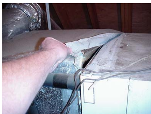
Figure 29 System with failed tape, and omitted fasteners, in USA [© Weldin Engineering]
