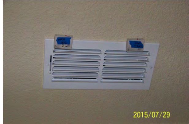
Figure 4 Methods used to monitor central forced air system use.
