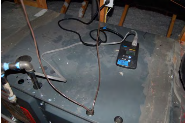
Figure 4 Methods used to monitor central forced air system use.
