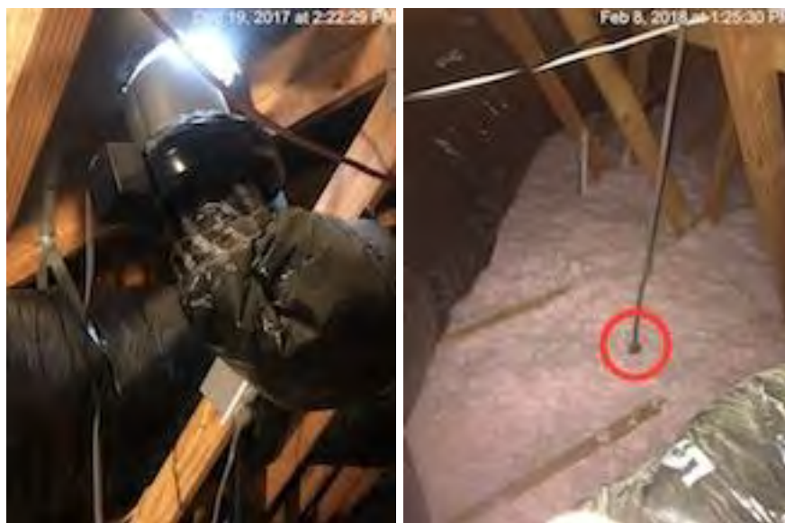
Figure 11: Continuous exhaust ventilation provided by a fan in attic
