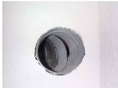
Picture 8: (Multi-Family Building) Connecting duct (flexible) with a strong leakage (the ATD has been removed, it was directly – and bad – mounted on the connecting duct)
