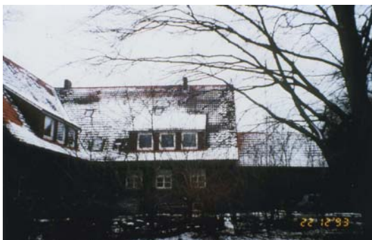
Figures 1+2: Thawed snow and the appearance of fog at 50 Pa pressurization show how air is flowing at the internal walls, beam ceilings and attic areas, and that there are energy losses in spite of the 200 mm insulation thickness.
