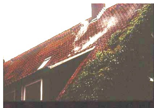
Figures 1+2: Thawed snow and the appearance of fog at 50 Pa pressurization show how air is flowing at the internal walls, beam ceilings and attic areas, and that there are energy losses in spite of the 200 mm insulation thickness.
