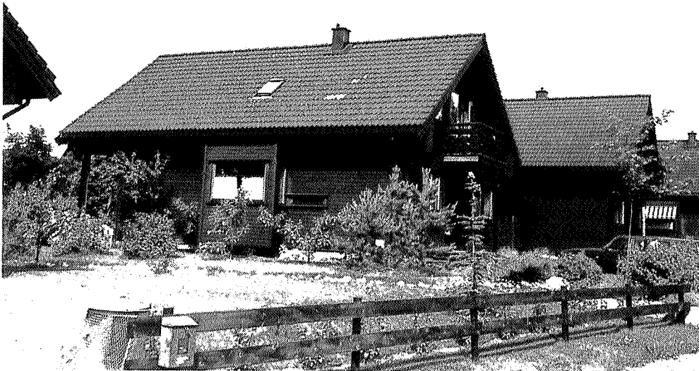
Figures 1 a and 1 b Views of the test houses
