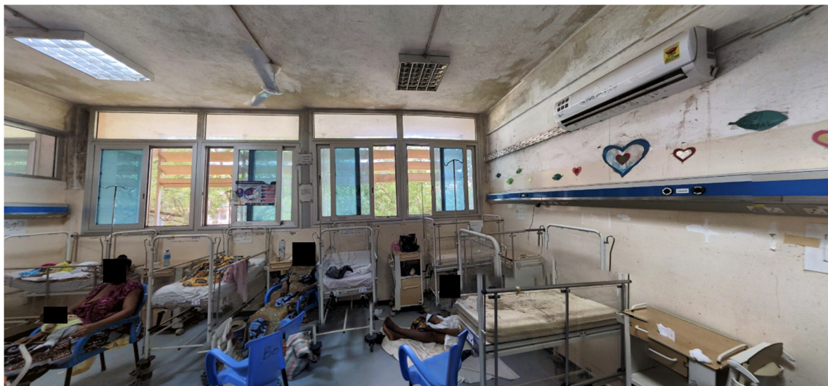
Figure 3: Ventilation openings and air-conditioning unit in the TH Paediatrics U6m ward. Sliding windows in lower portion and fixed glazed units in upper. External shading to windows is visible.
