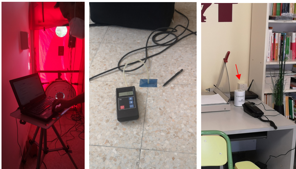
Figure 2: a) Airtightness test with blower door equipment; b) Differential pressure measurements between the internal environment and the ground; c) Continuous radon monitoring equipment
