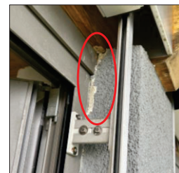
Cracks in the plaster inside and outside
