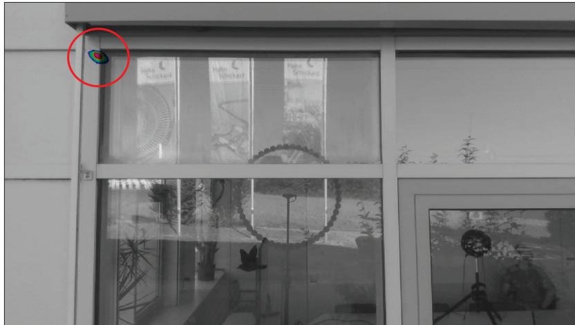
Hole in window seal
