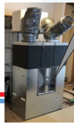
Figure: Desiccant unit
