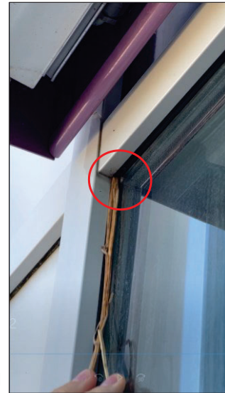
Hole in window seal
