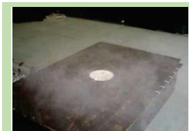
Displacement Flow Type Diffuser *)
