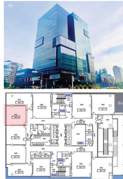
Zone description and test setup at Longueuil campus, University of Sherbrooke
