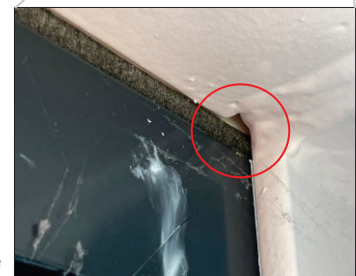
Tilt window and hole in steel structure
