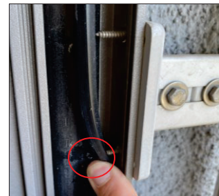
Window seals are damaged
