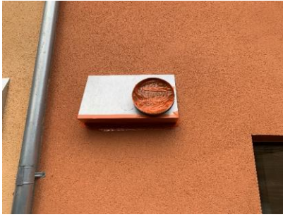
Figure 3: MVHR inlet and exhaust sealed both internally and externally
