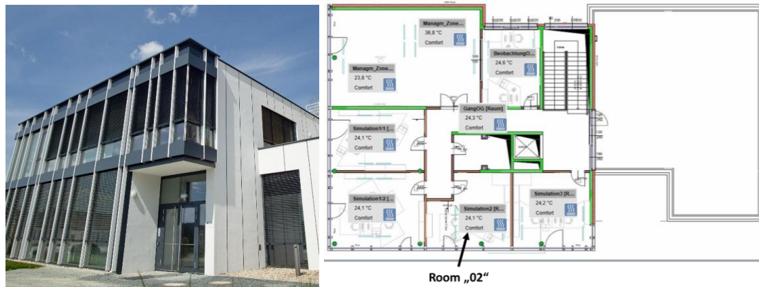
Figure 4: Left: Picture of the south-south-east façade of the case study building “Energetikum”. Right: Upstairs floorplan with investigated room “02”. Source: Forschung Burgenland.
