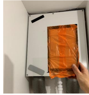
Figure 3: MVHR inlet and exhaust sealed both internally and externally
