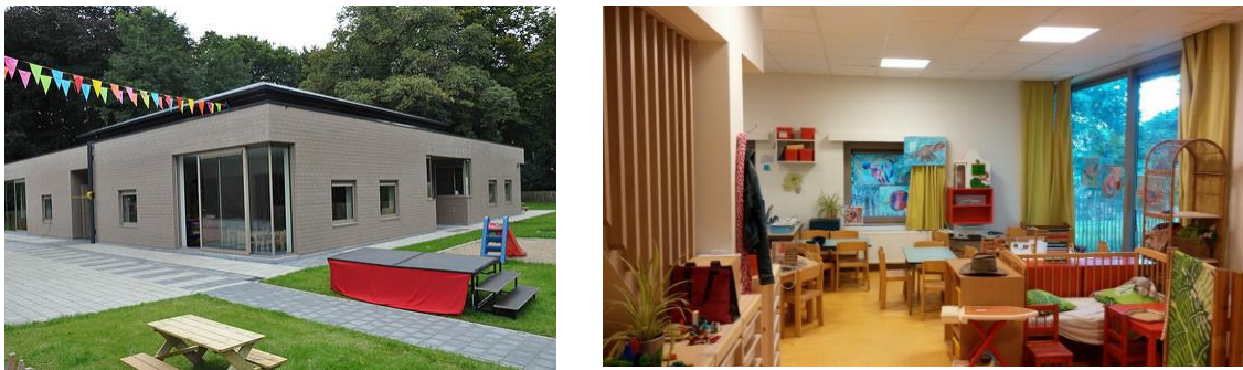
Figure 1. left) View of south-east façade of the kindergarten “De Boomhut”, right) interior of the classroom measured
