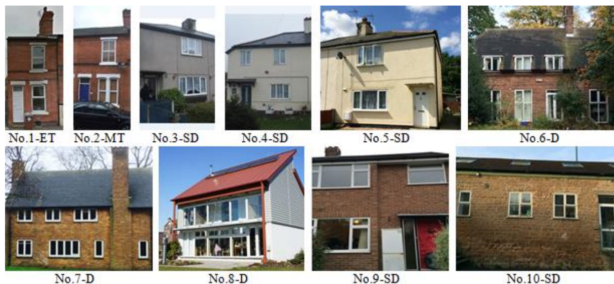
Figure 1 Test houses (D: detached; SD: semi-detached; ET: end-terraced; MT: Mid-terrace)
