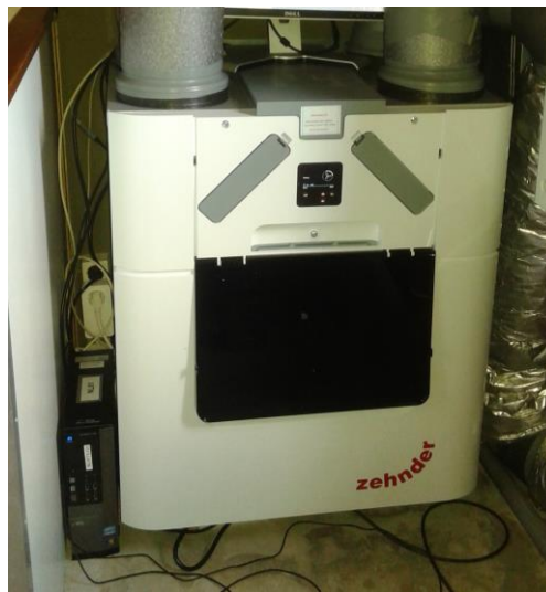
Figure 1: Photograph of the ventilation unit with a heat exchanger in the house in The Netherlands.
