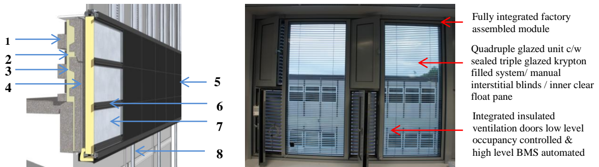
Figure 3: (a) Opaque Retrofit module, (b) fenestration module (including ventilation inlets)
