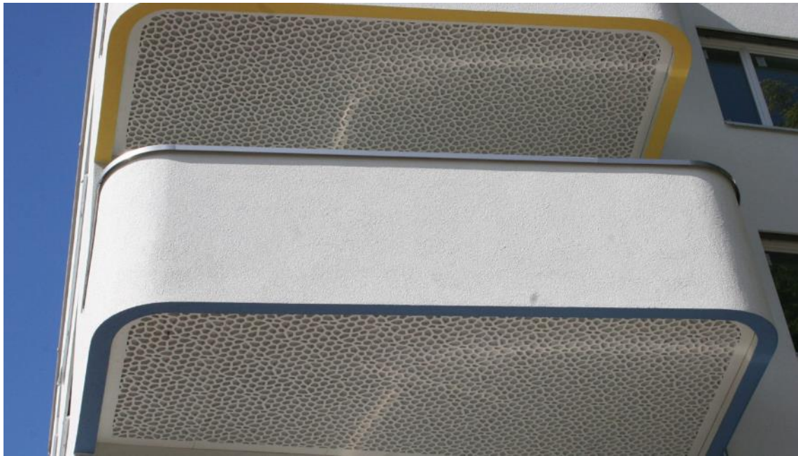
Figure 4: Absorptive lining to the underside of a balcony
