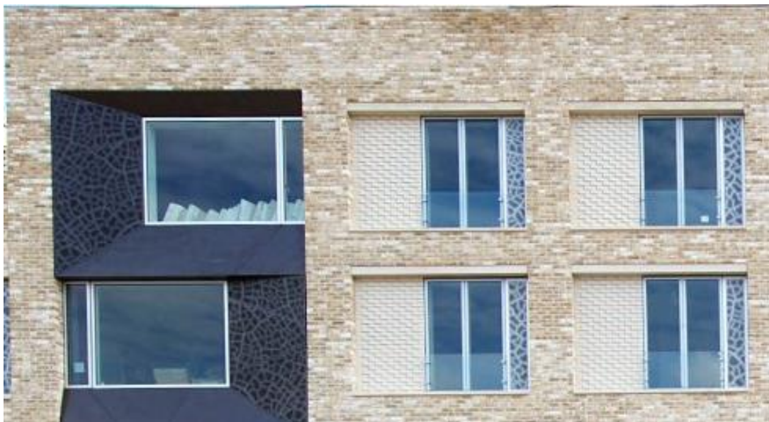
Figure 7: Lot 5 façade showing perforated panels adjacent to windows
