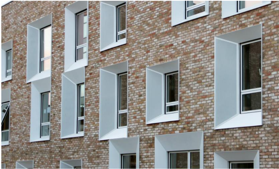
Figure 6: Lot 3 façade showing perforated panels to window reveals
