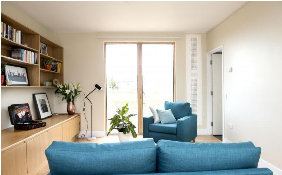
Figure 8: Internal view of attenuated vent opening adjacent to the windows
