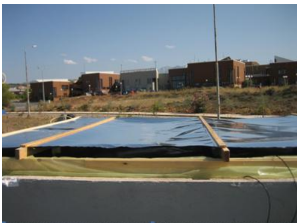
Figure 1: Wooden frame is the pond's perimeter. Figure 2: Nylon for pond waterproofing and floater.
