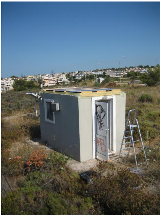
Figure 5: Photo of the building with the investigated pond on the roof.
