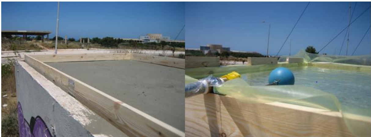
Figure 1: Wooden frame is the pond's perimeter. Figure 2: Nylon for pond waterproofing and floater.
