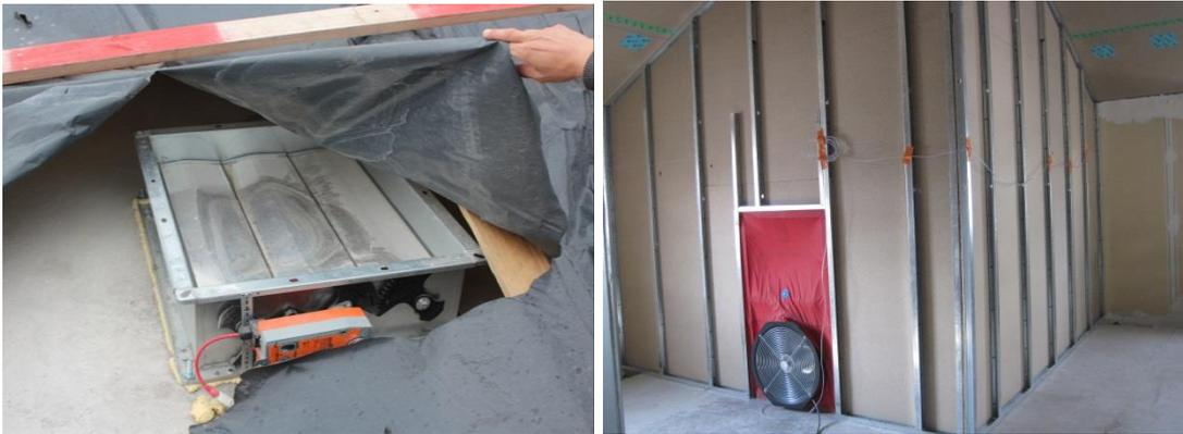
Figure 4: Motorized grill for ventilation shaft - Figure 5: intermediate testing in a corner of the top floor
