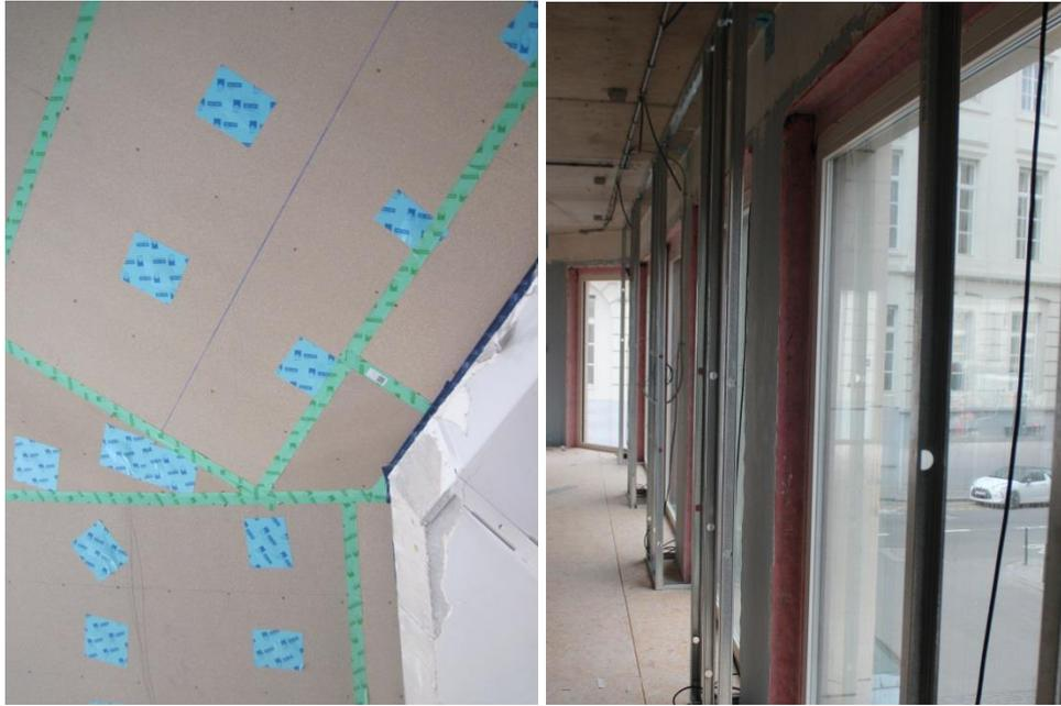
Figure 2: Airtightness tapes on the panel joints - Figure 3: Membranes around window frame edges
