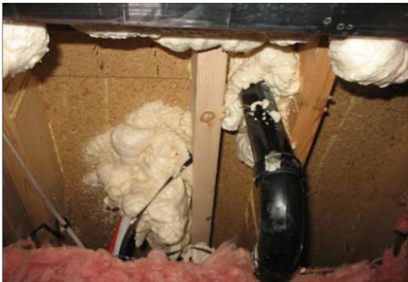
Drain and water lines after sealing
