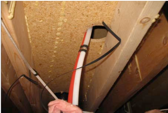
Water line in floor (from below)
