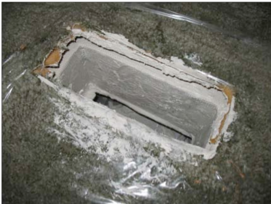
Floor register (from above) after sealing with mastic
