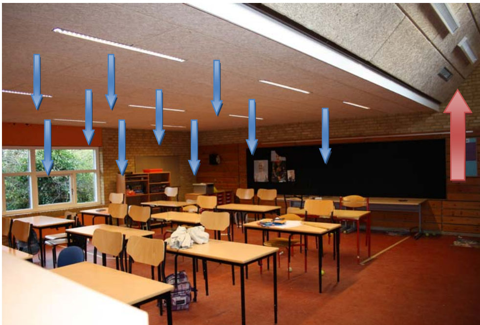
Figure 2. Picture of room 42 with principal airflow pattern of the diffuse ceiling inlet indicated with arrows.
