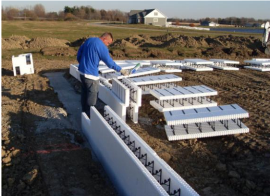
Figure 2 ICF (Insulated Concrete Form) foundation wall used for Equinox perimeter.
