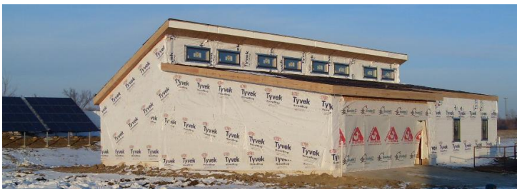
Figure 7 Completed SIPs panel installation with house wrap and windows installed.
