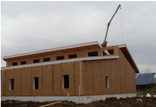
Figure 6 Installation of SIPs roof panels on Equinox.
