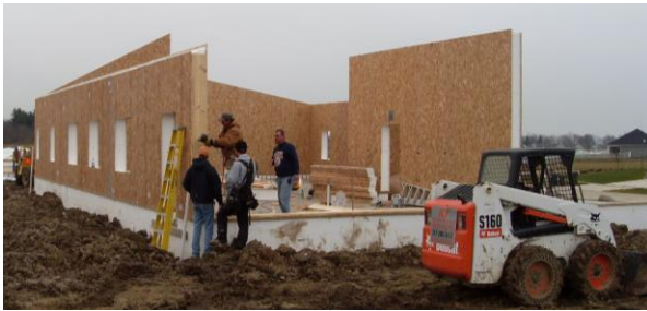
Figure 5 Continued placement of SIPs wall panels around the house perimeter.
