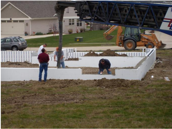
Figure 3 Concrete poured in ICF foundation wall.
