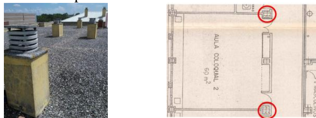
Fig.5 left) Cross ventilation in an Andalusian school. Right) Natural Ventilation system in an Andalusian school built in 1985
