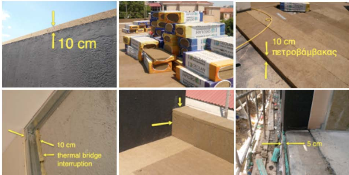
Figure 4. Outside thermal insulation with minimised thermal bridges is composed mostly by 10 cm rockwool. Foundations are insulated with 5 cm xps. In some special cases it was necessary to use internal thermal insulation with 10 cm rockwool.
