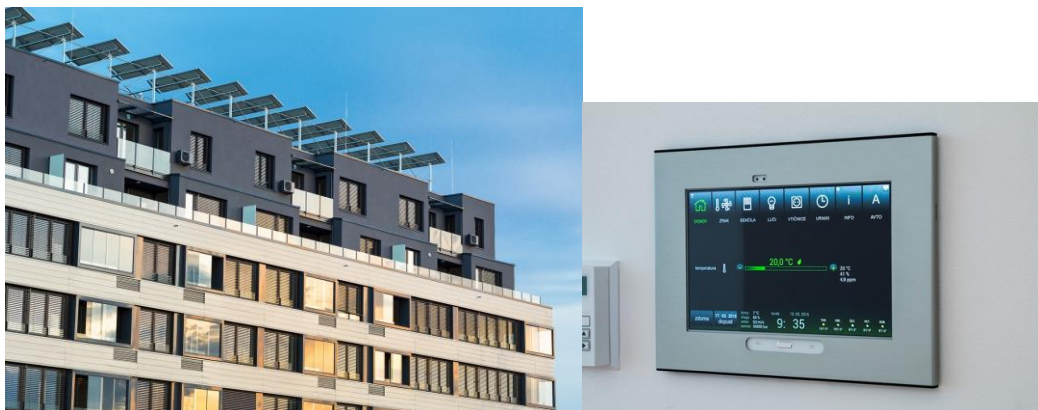
Figure 2: Eco-Silver House – PV power plant on the flat roof and the intelligent control unit in each apartment (Photo: Borut Slabe).
