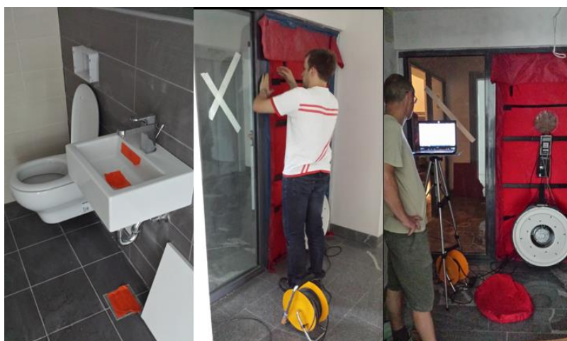
Figure 6: Preparation and execution of Blower door tests.
