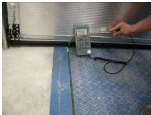
Figure 7: Detail, movable loading bridge with integrated sealing. A clearly visible air leakage only remains at door level.
