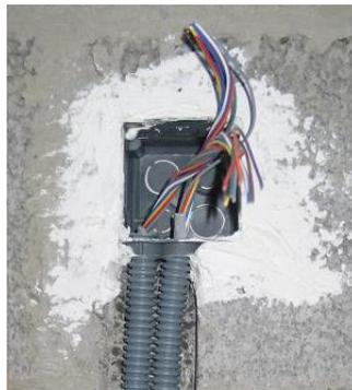
Figure 6: electrical outlet encased in a wall<sup>1</sup>
