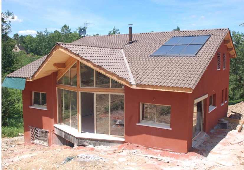
Figure 1: View of the south façade of the building
