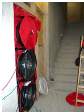
Figure 5. BlowerDoor MultipleFan (3 fans) in the stairwell
