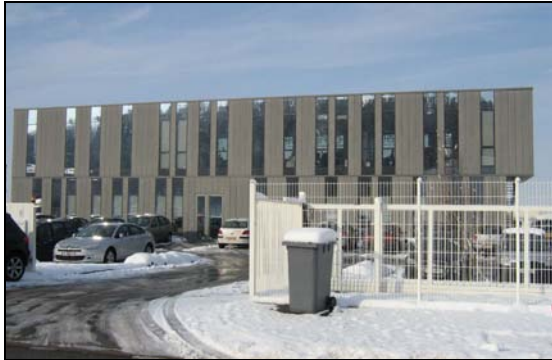
Figure 1 : Outside view of the office building
