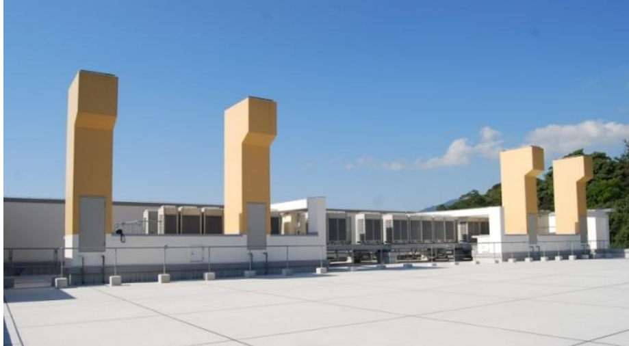
Fig.8 Appearance of chimney (Model F) in real building
