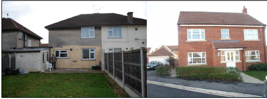
Figure 3. Rear of a semi-detached house in Doncaster (left) and a single family detached house in Yorkshire (right).
