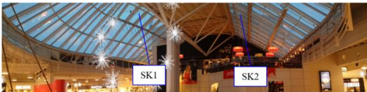
Figure 2: Skylights in the central atrium and the cafeteria located on the mezzanine below. Openable windows are present on both sides of the skylight.
